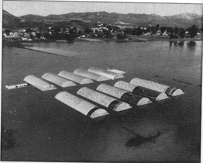
A hydroponics garden under floodwaters at Lake Elsinore as seen from helicopter.
