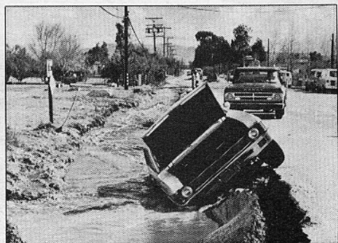
Floodwaters have torn away pavement on Old Magnolia Avenue.
