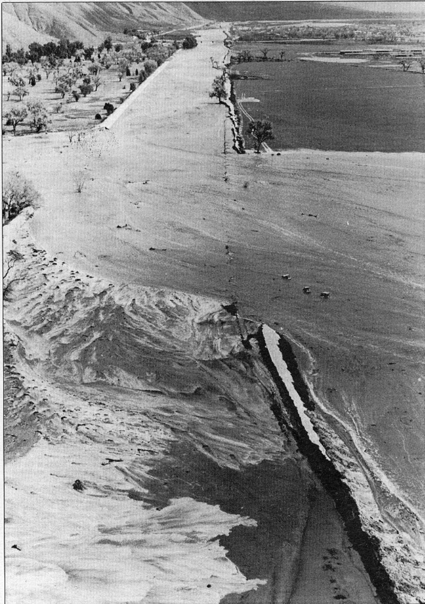
A break in the northern San Jacinto River levee has caused flooding in the Hemet area.
