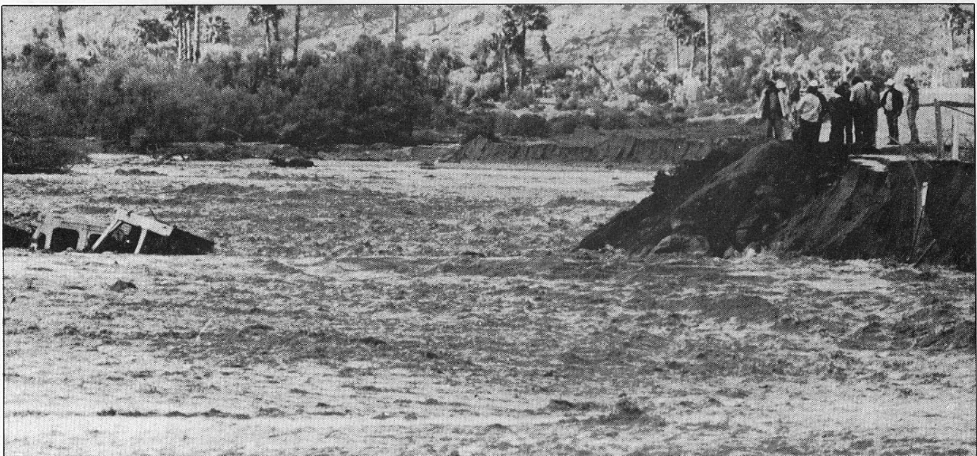
Two pieces of heavy construction equipment lie nearly submerged (left) in Palm Canyon Wash in Palm Springs following a levee break yesterday.
