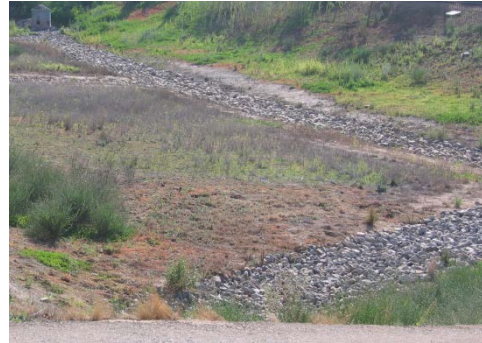
Figure 3: Gravel filled low-flow trench
