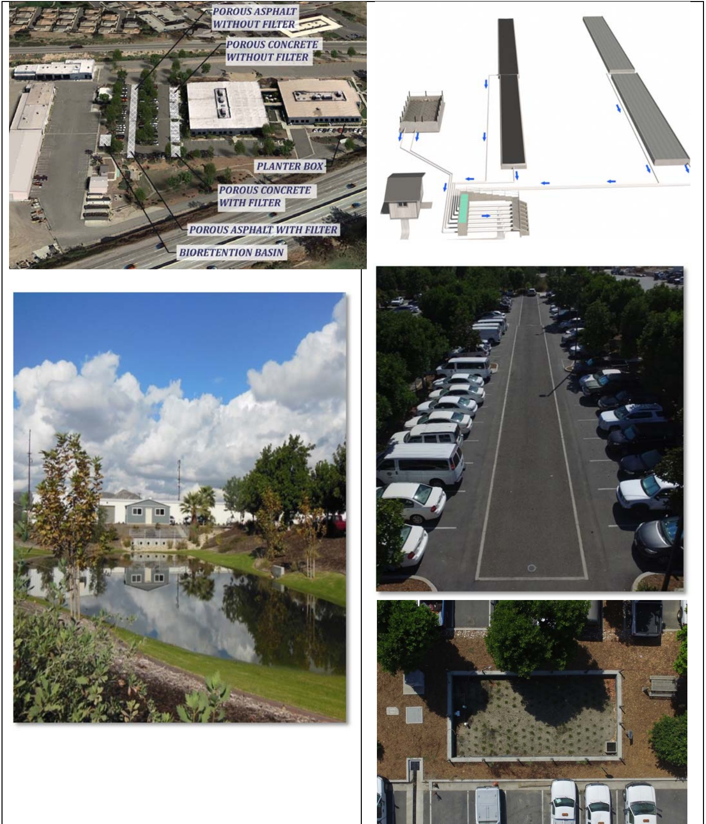
Figure 4-2: Photographs of the LID Integrated Management Plan Testing and Demonstration Facility
