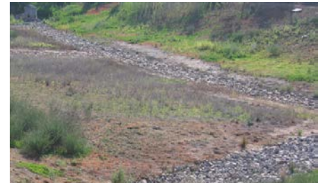
Gravel filled low-flow trench
