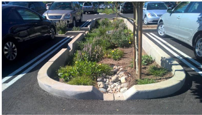
Figure 2: Example Curb Cut
