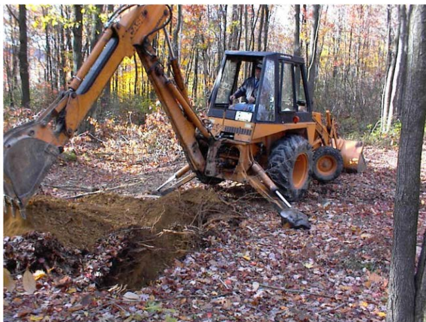
Photo 9 – Test Pit Excavation
