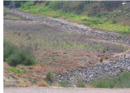
Figure 3: Gravel filled low-flow trench
