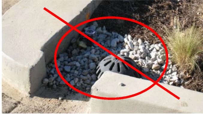
Figure 6: Incorrect Placement of an Overflow Inlet
