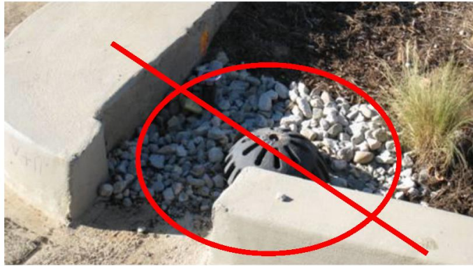
Figure 5: Incorrect Placement of an Overflow Inlet
