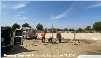
Pouring Concrete Footings: September 17, 2020
