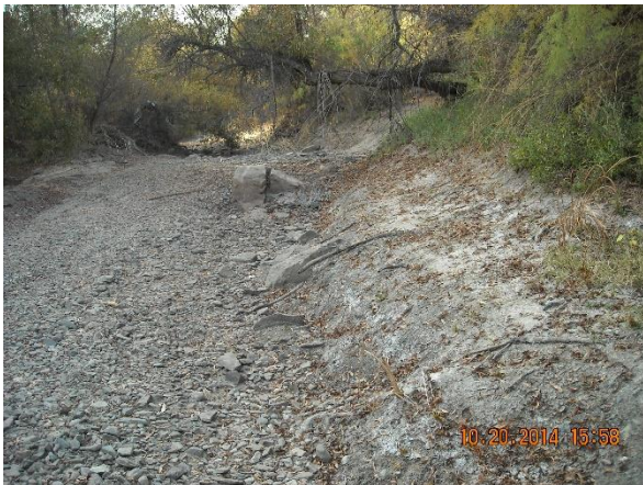
Coarse material along low-flow channel invert
