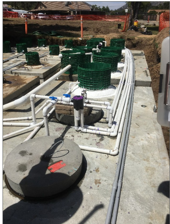
Figure 2-31. Advanced Treatment Septic System at Rainbow Oaks Restaurant
