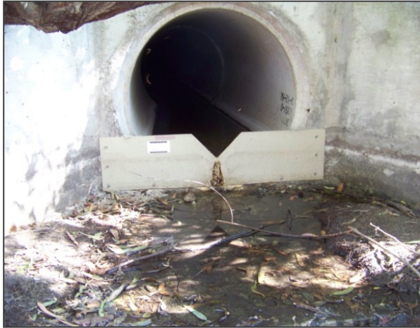
Figure 2-25. Example Flow Meter and Weir Installation
