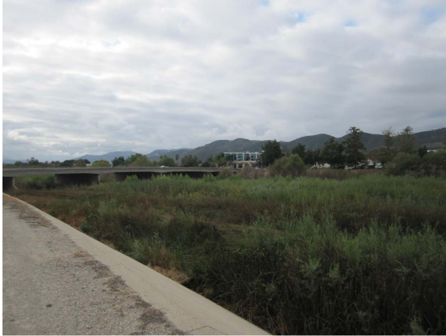
Figure 4-21. Looking downstream near the Murrieta Creek and Santa Gertrude Creek confluence. Heavily vegetated channel bed and concrete side slope.
