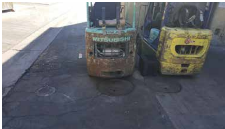
Stains from grease near interceptor
