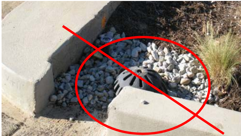
Figure 6: Incorrect Placement of an Overflow Inlet.
