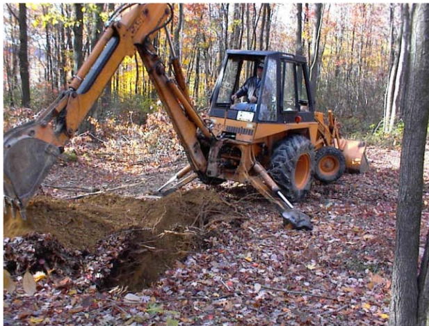
Photo 9 – Test Pit Excavation
