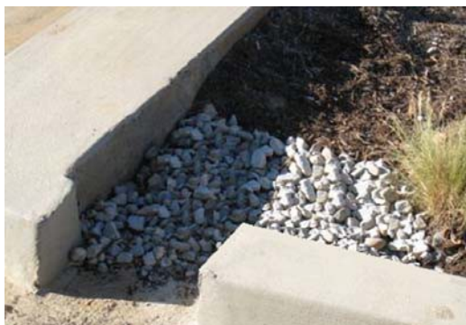
Figure 2: Curb Cut located in a Bioretention Facility
