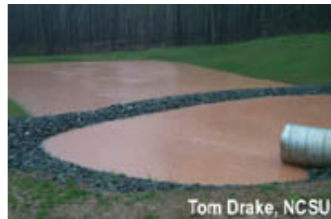
Figure 2: Forebay filled with stormwater
