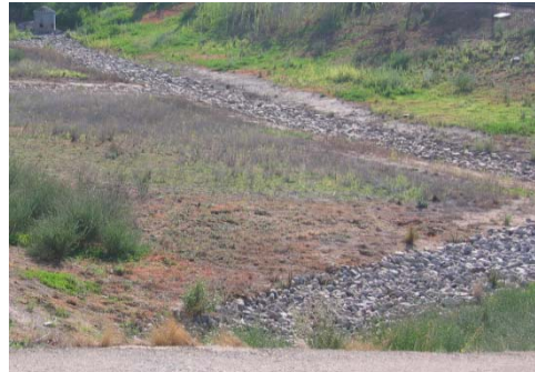
Figure 3: Gravel filled low-flow trench
