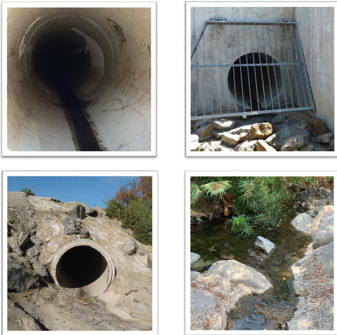
Figure 3-1. Storm Drain Outfalls during Dry Weather Monitoring
