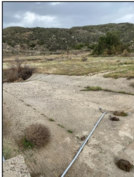
Figure 7. Wilson Creek Channel on 3/11/2020 (looking downstream)
