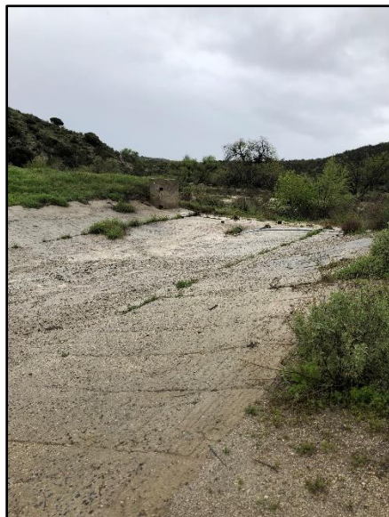
Figure 8. Wilson Creek Channel on 4/10/2020 (looking upstream)
