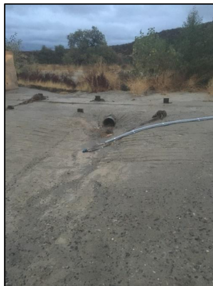
Figure 4. Wilson Creek Channel on 11/21/2019 (looking upstream)
