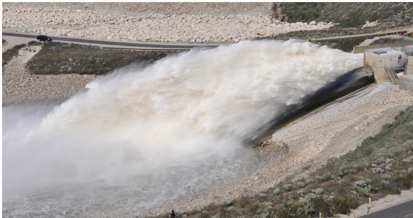
ABOVE: The Corps conducting a routine test of the outlet structure at Seven Oaks Dam.
