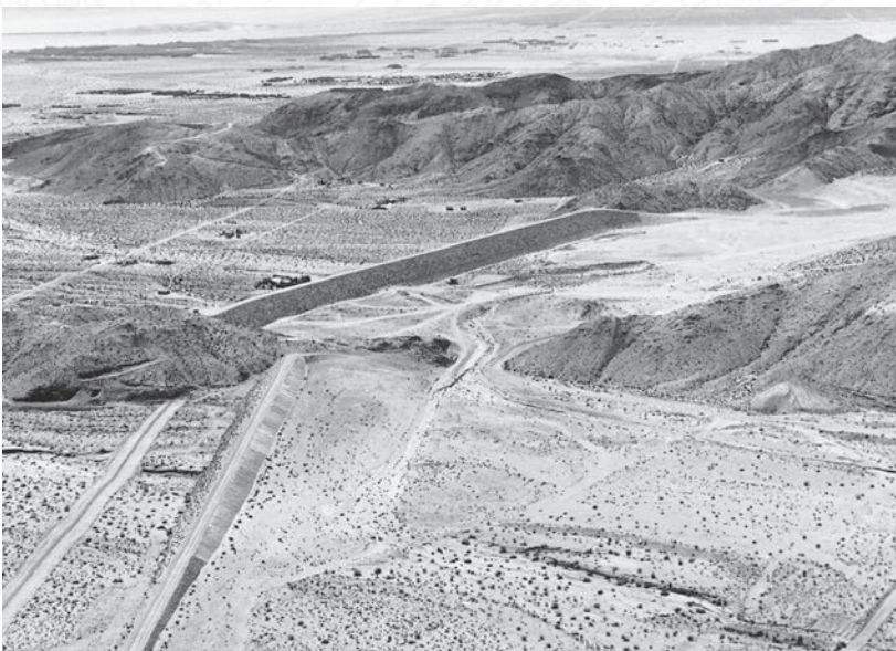
LEFT: At its construction in 1968, Wide Canyon Dam east of Desert Hot Springs was the largest of the District dams. Wide Canyon Dam is 2,225 feet long, 67 feet high, and contains 664,000 cubic yards of earth and rock fill. Several times in its history, Wide Canyon Dam has prevented flooding downstream mainly from flash flooding in the summer time.
