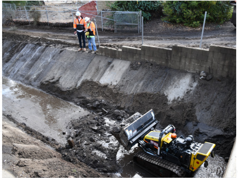
ABOVE: The District partnered with other agencies to clean up the debris in Lake Elsinore after the 2019 storms. This photo shows a remote controlled bulldozer cleaning debris from a low clearance box culvert.
