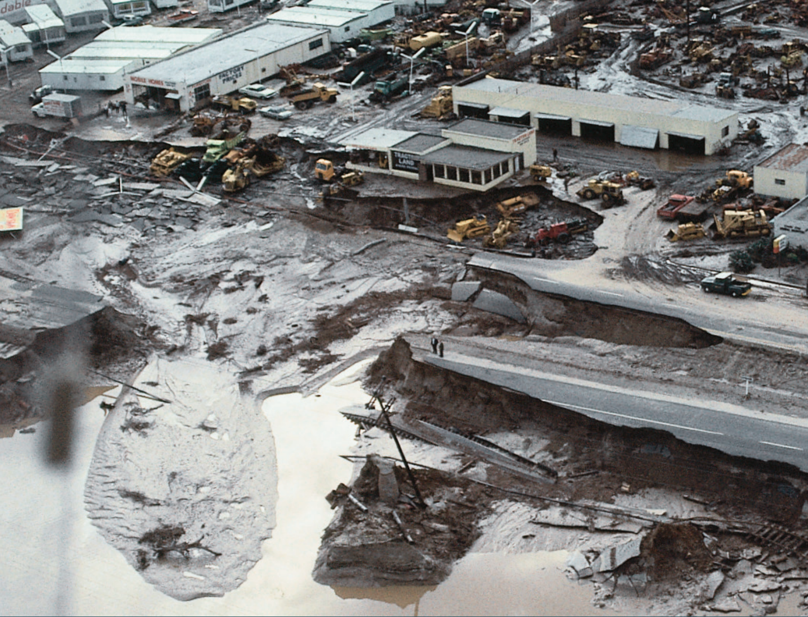
ABOVE: Aftermath of the storm of February 1969 flooding on Temescal Creek impacting Magnolia Avenue and the Pacific Electric Railroad tracks in Corona. This problem was corrected by the construction of Temescal Creek Channel.
