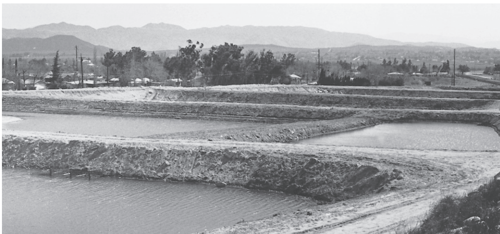
LEFT: Little San Geronio Creek Spreading Grounds, typical of several facilities operated by the District. Minor storm flows are turned out of the main stream into basins where the water percolates to groundwater. This facility is still in use conserving floodwater.
