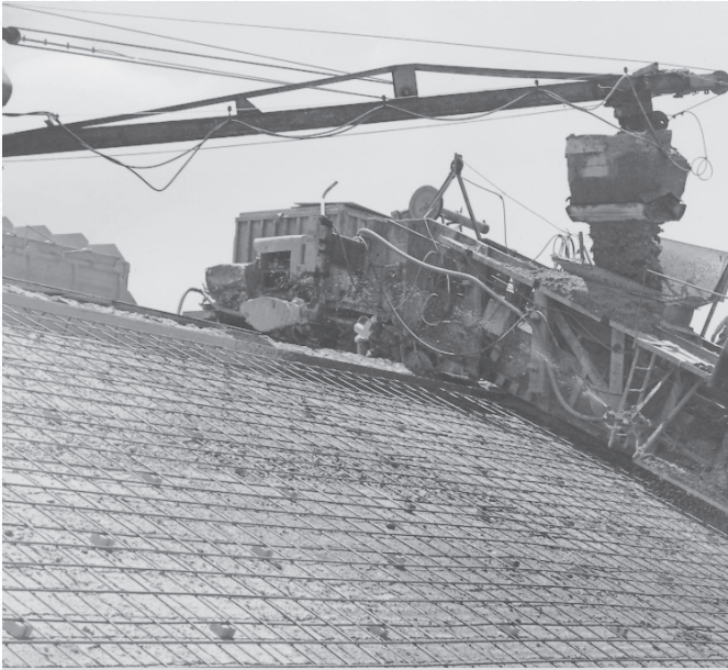
ABOVE: Slope-paving on Bautista Creek Channel, June 1961. Bautista Creek Channel was a major project for the District and helped manage a major flooding problem in the Hemet area.
