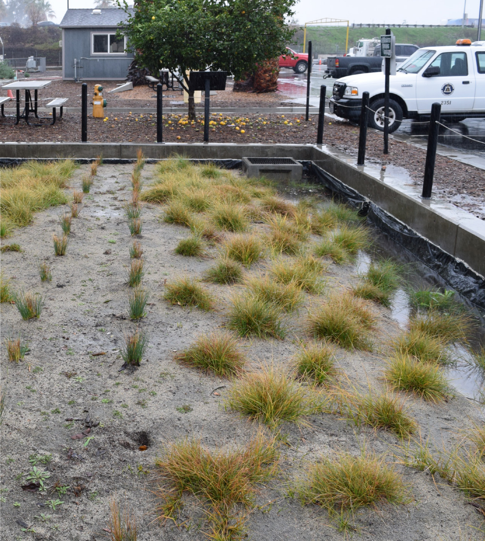
ABOVE: LID Bioretention Basin; this is one of the most commonly used LID BMPs in southern California and elsewhere. The structure in the background is the LID Data Collection Center.
