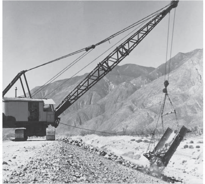
ABOVE: Placing rock "revetment" on the San Jacinto River Levee during its construction by the U.S. Army Corps of Engineers in 1961.
