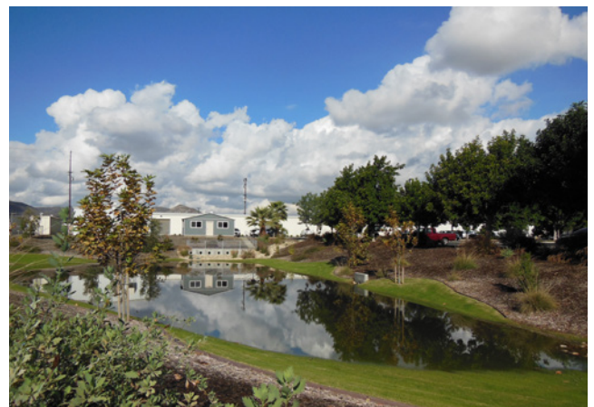
ABOVE: The Infiltration Basin (also known as Lake Smithhammer) located on-site is an example of a LID BMP.
