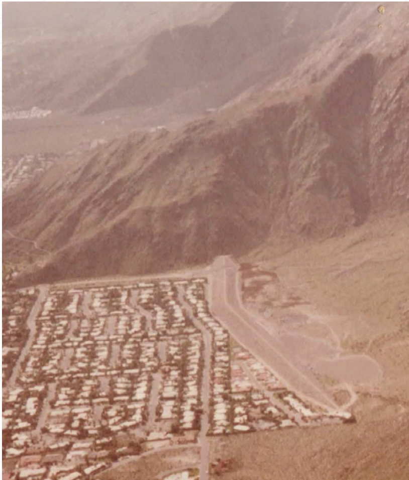
ABOVE: Tachevah Dam, Palm Springs. This earth fill dam which was constructed by the U.S. Army Corps of Engineers in 1964 protects the northern and downtown areas of Palm Springs.
