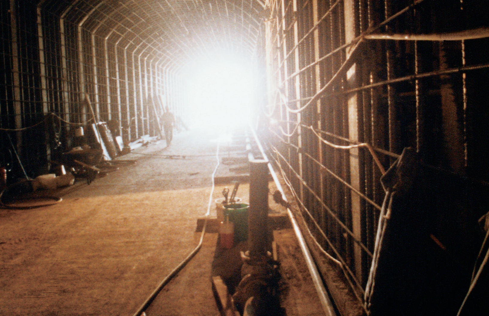
ABOVE: Construction inside the Oak Street Channel culvert under the 91 Freeway in Corona. This structure was constructed using micro-tunneling techniques.
