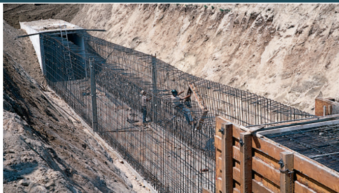
ABOVE: Magnolia Center Storm Drain, another 1970 bond issue project, drains a highly urbanized area in Riverside. Construction of an open channel was not practical and, therefore, the system is all underground. Shown here is a section of reinforced concrete box culvert being formed and reinforcing steel being placed.
