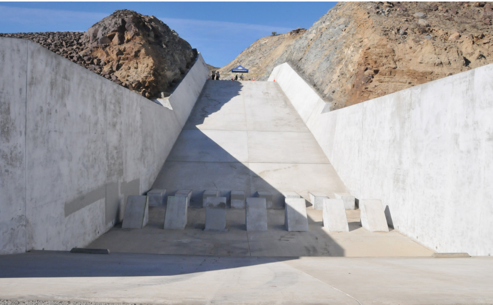
ABOVE: This photo shows Eagle Canyon Dam's spillway shortly after construction. The spillway was constructed through a hillside of fractured rock and an inactive seismic fault. To stabilize the hillside prior to the construction, tie-backs were installed.
