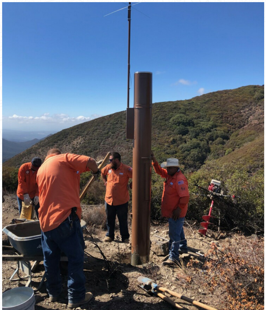
ABOVE: District Operations and Maintenance crews assist with the installation of a new real-time rain gauge to assist in emergency planning and safety evacuations in the Holy Fire area.
