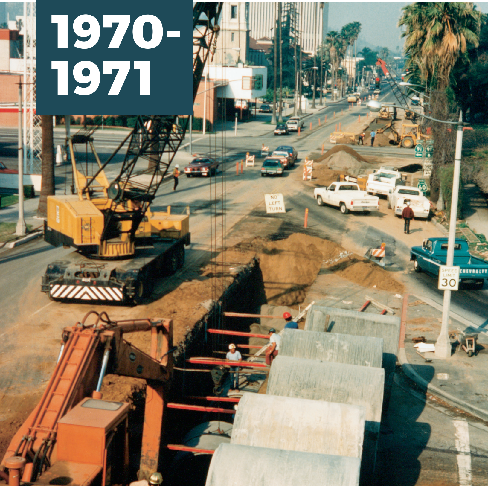
ABOVE: Placing 102" diameter reinforced concrete pipe on 7th Street in Riverside, looking westerly from the 91 freeway. The Box Springs Drain was a major 1970 bond issue project.
